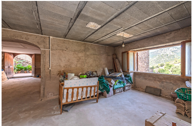
House 2 (bare brickwork)
