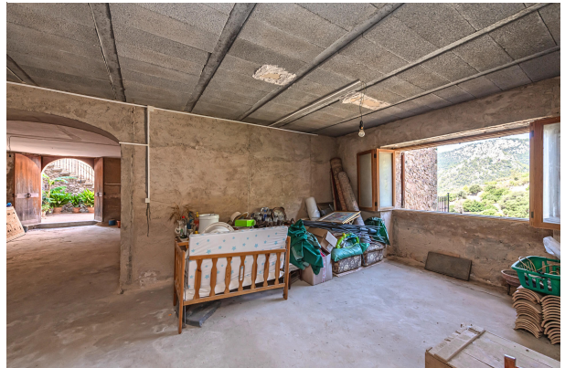
House 2 (bare brickwork)
