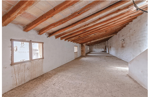
New wing (attic)
