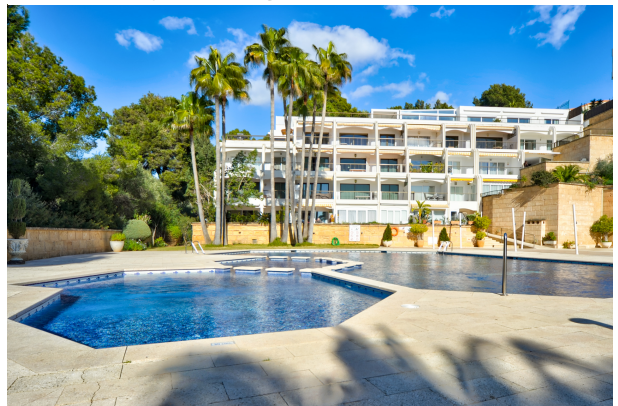
3. Community swimming pool in Portals
