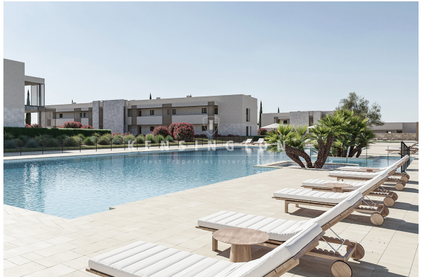
Complex and pool
