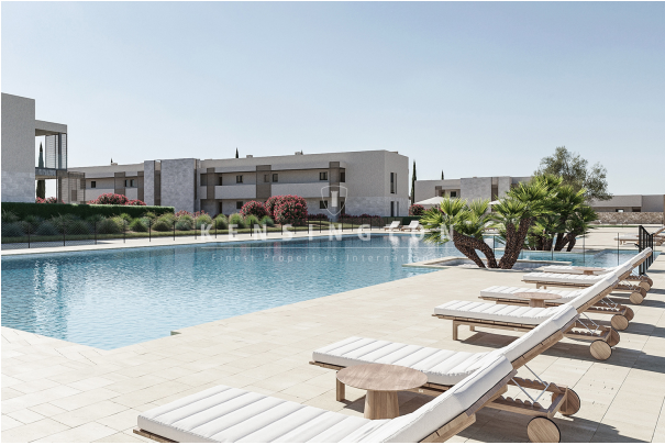
Complex and pool
