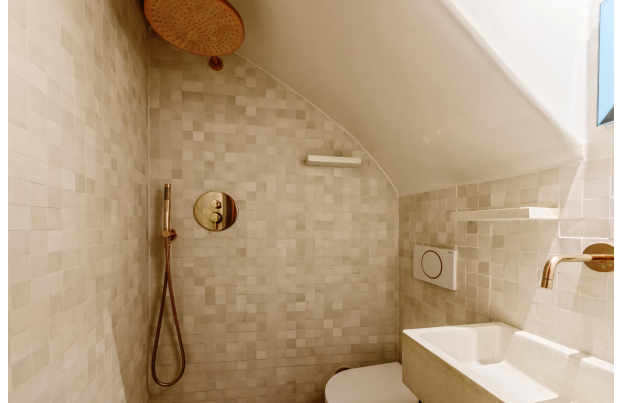
Ground floor bathroom
