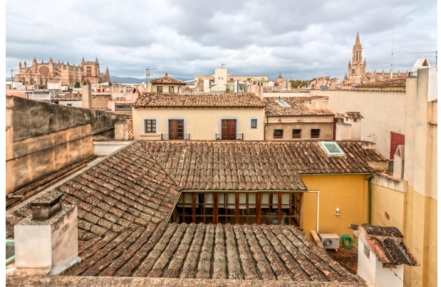
View rooftop terrace
