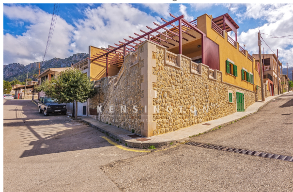
Beach house in Port des Canonge house facade
