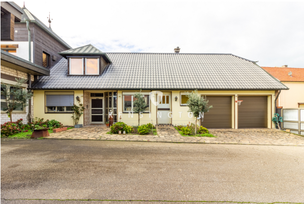
KSW517-Haus in Bellheim
