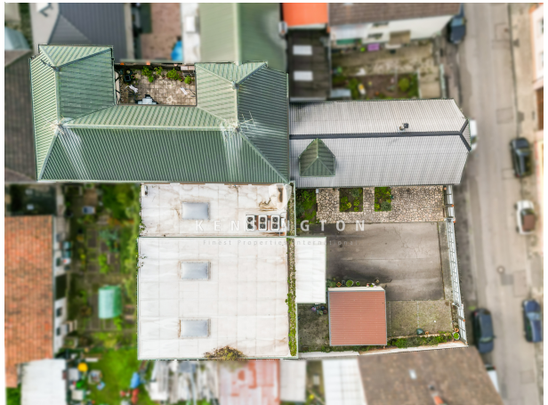
KSW517-Haus in Bellheim
