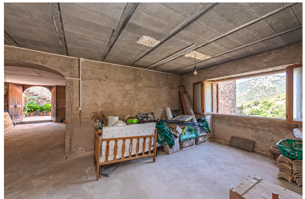
House 2 (bare brickwork)
