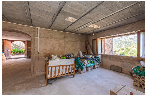
House 2 (bare brickwork)
