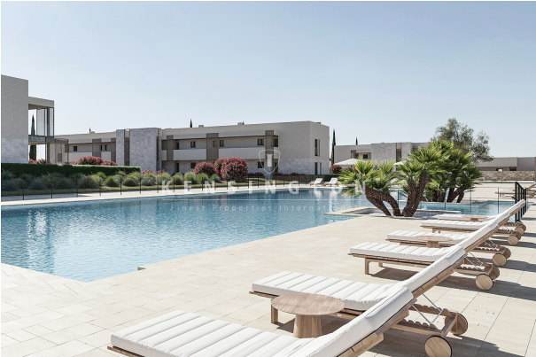
Complex and pool
