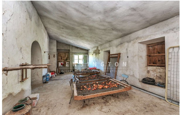
Farm house - Roof truss
