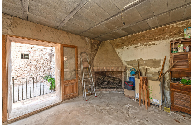
House 2 (bare brickwork)
