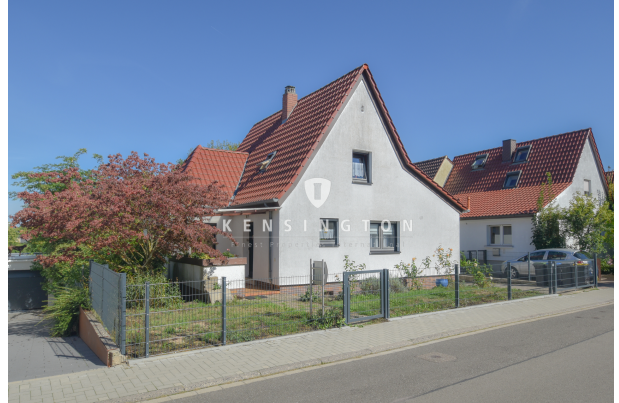
KSW504-Haus in Landau
