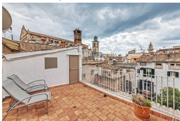
Communal rooftop terrace
