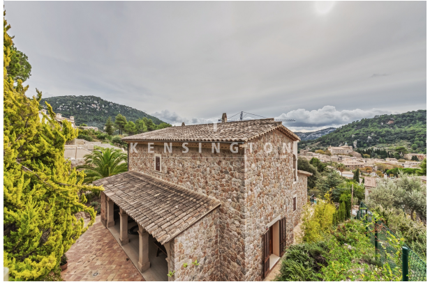
View garden above house
